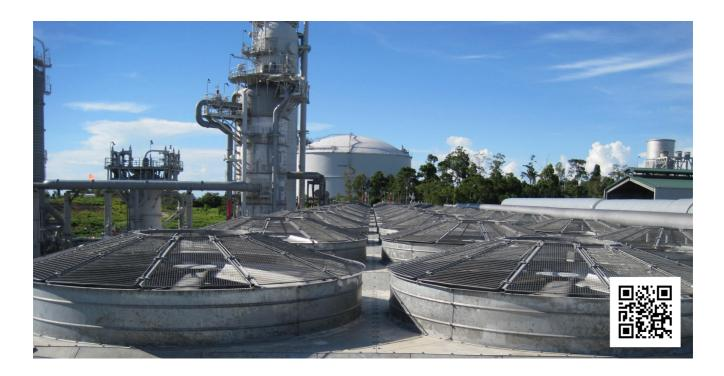
The production of LNG in liquefaction plants is limited by the output pressure of the propane compressor. This is directly linked to the efficiency of the propane condenser, desuperheater and sub-cooler. The performance of these air coolers decreases greatly with the ambient temperature.
