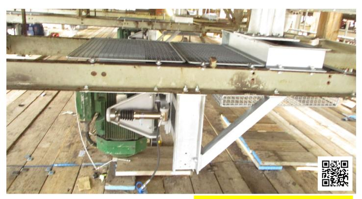
In 2019, Kelvion Thermal Services completed an airside revamp of a Kerosene Product Cooler in the Crude Distillation Plant of a UK refinery. The Kerosene Product Cooler had a higher than design outlet temperature, this is due to the old, fouled and inefficient equipment.
